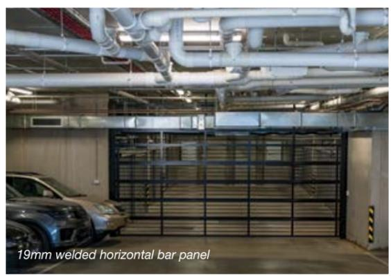
19mm welded horizontal bar panel
